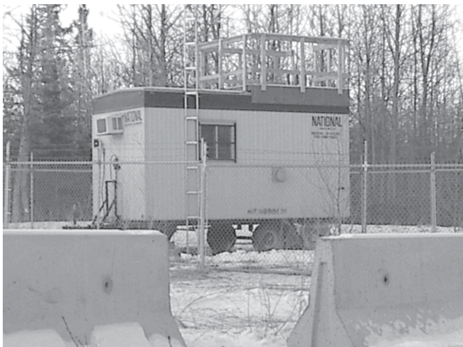
The new WCAS air monitoring station at Hinton.
